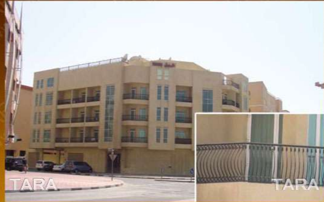
G+4 Floor Res/Comm Bldg at Al Hudaiba - Balcony Railing
