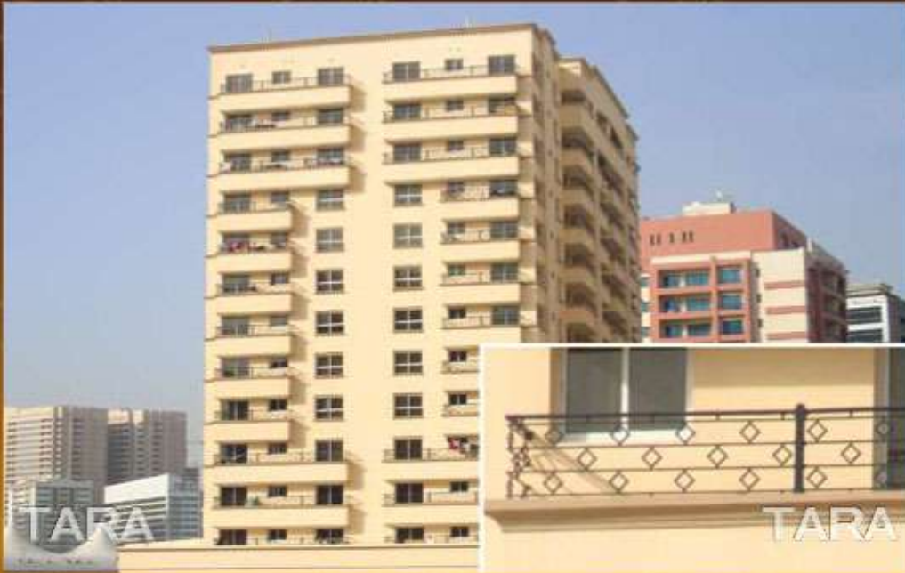
G+12 Floor Res/Comm Bldg at Al Nahda - Balcony
