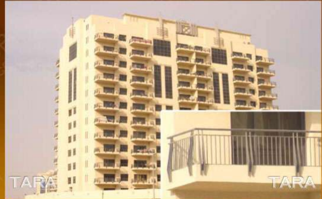
G+11 Floor Res/Comm Bldg at Sharjah - Balcony
