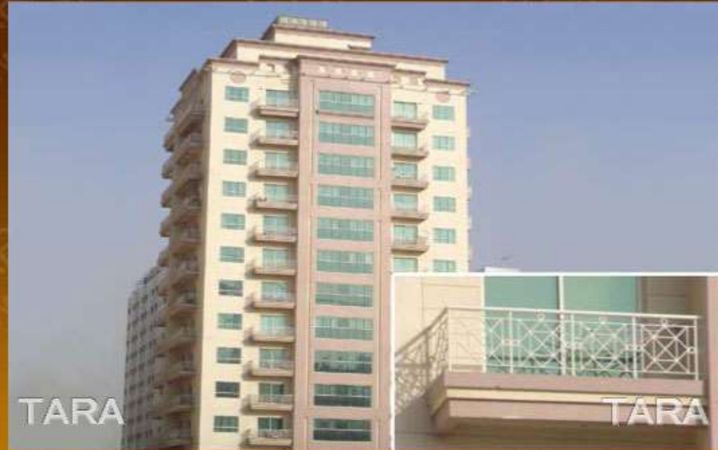
G+11 Floor Res/Comm Bldg at Al Nahda - Balcony
