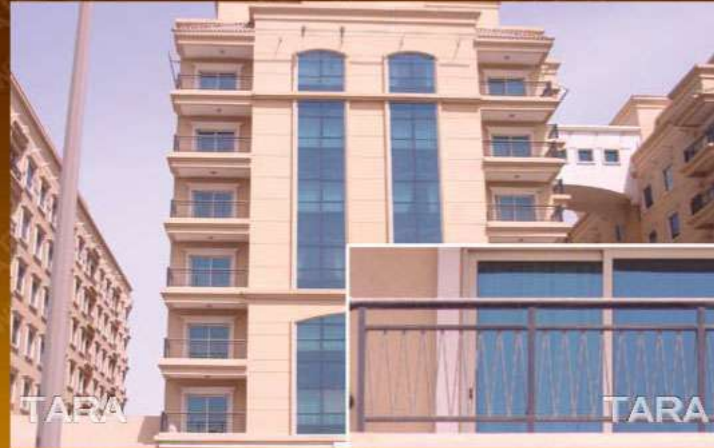
G+7 Floor Res/Comm Bldg at Al Nahda - Balcony
