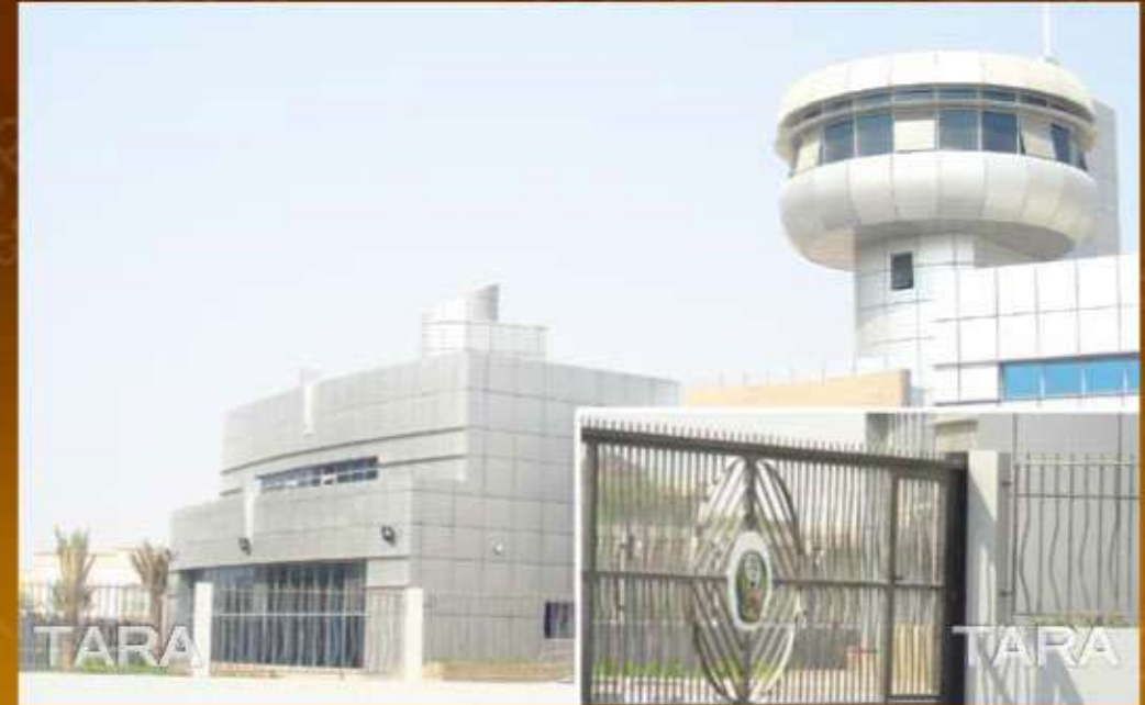
Dubai Municipality at Al Barsha - Gate & Fencing
