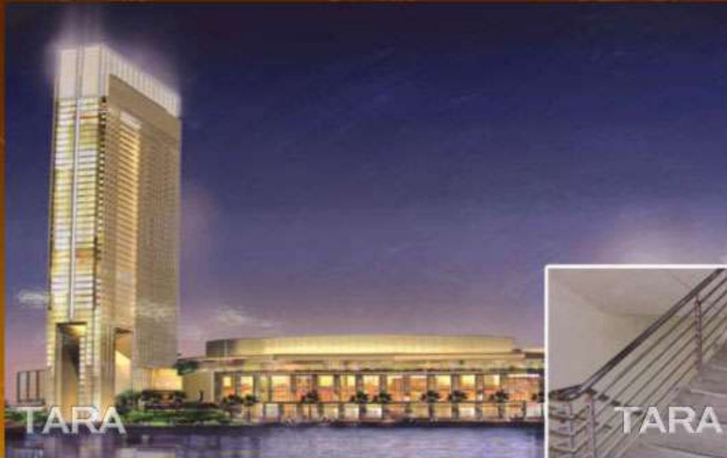
Dubai Marina Mall - Staircase Railing
