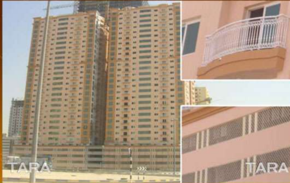
G+5P+25 Floor Res/Comm Bldg, Al Nahda Area - Balcony, Parking Grills
