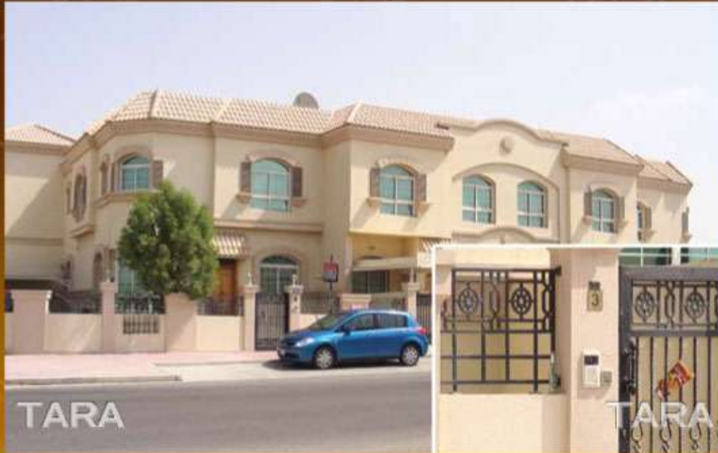
12 Villas at Mirdiff - Gates, Staircase, Fencing
