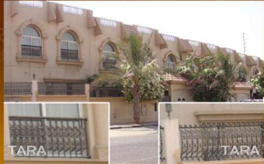
12 Villas at Mirdiff - Gates, Fencing, Balcony, Parapet, Swimming Pool
