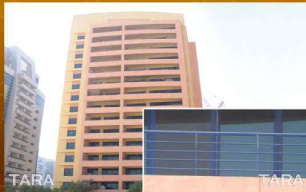
G+14 Floor Res/Comm Bldg at Al Nahda - Balcony
