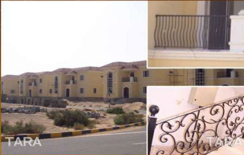
34 villas at Sharjah - Gates, Staircases & Balcony
