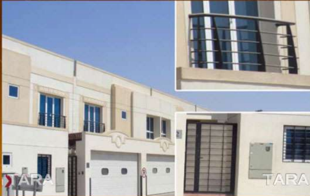
14 Villas at Al Hudaiba - Gates, Fencing
