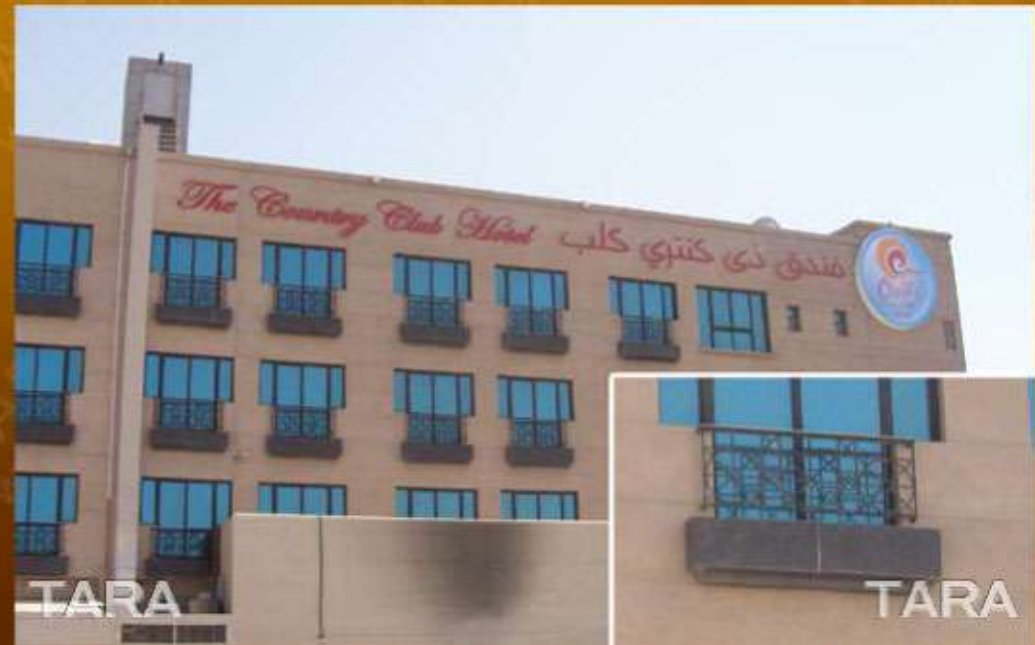
G+3 Floor Res/Comm Bldg at Al Hudaiba - Balcony, Wall Mounted, Grills
