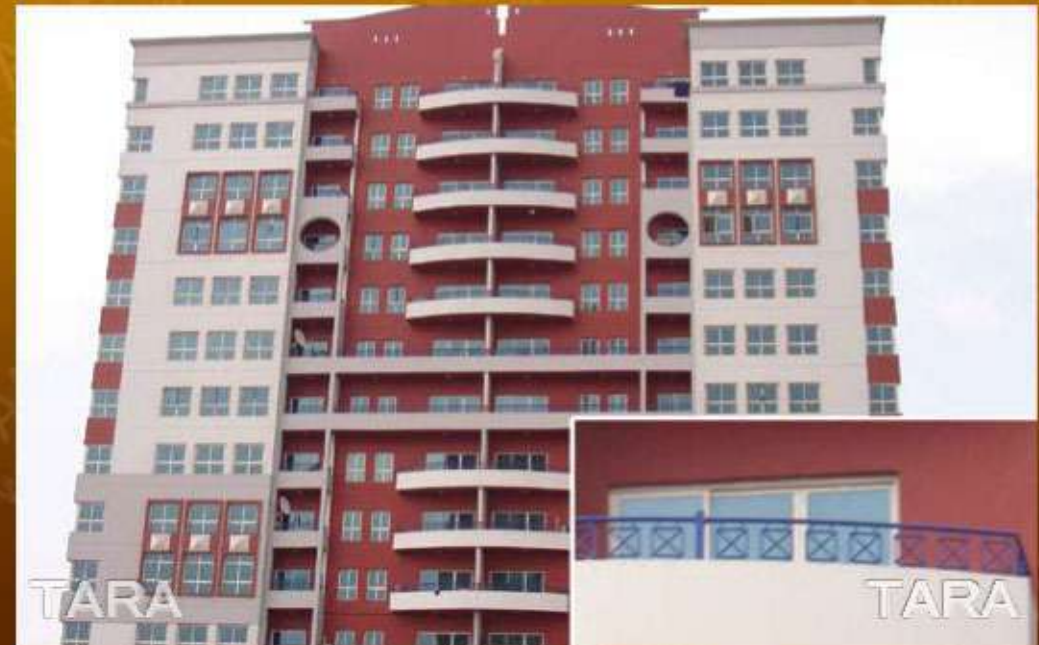
G+13 Floor Res/Comm Bldg at Al Nahda - Balcony
