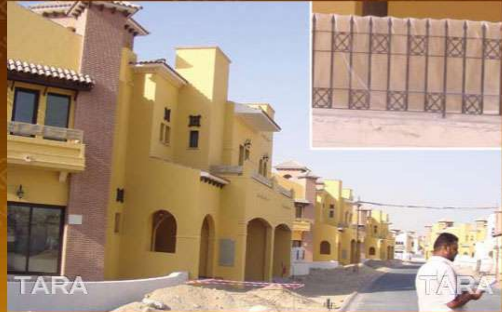
375 Villas at Mirdiff - Fencing & Gates
