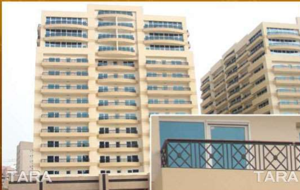
2B+G+12 Floor Res/Comm Bldg at Al Nahda - Balcony
