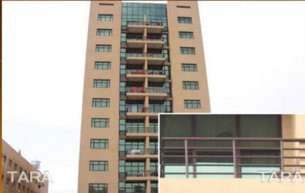
G+10 Floor Res/Comm Bldg at Al Nahda - Balcony
