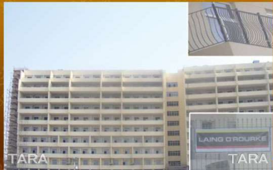
Motorcity Phase I at Motorcity - Gates, Fencing & Balcony
