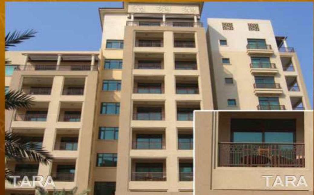
14 B+G+7 Floor Res/Comm Bldg at The Greens - Balcony
