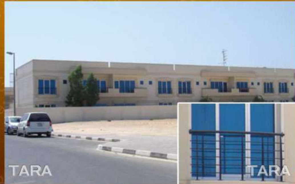
40 Villas at Al Hudaiba - Balcony
